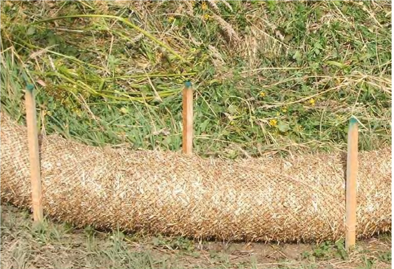
STRAW WATTLE – SHALLOW SLOPE ( \leq 4:1 ) (ALTERNATE STAKING)
